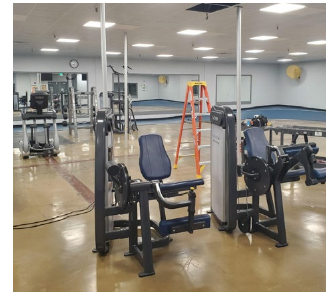
Above photo: During renovation
